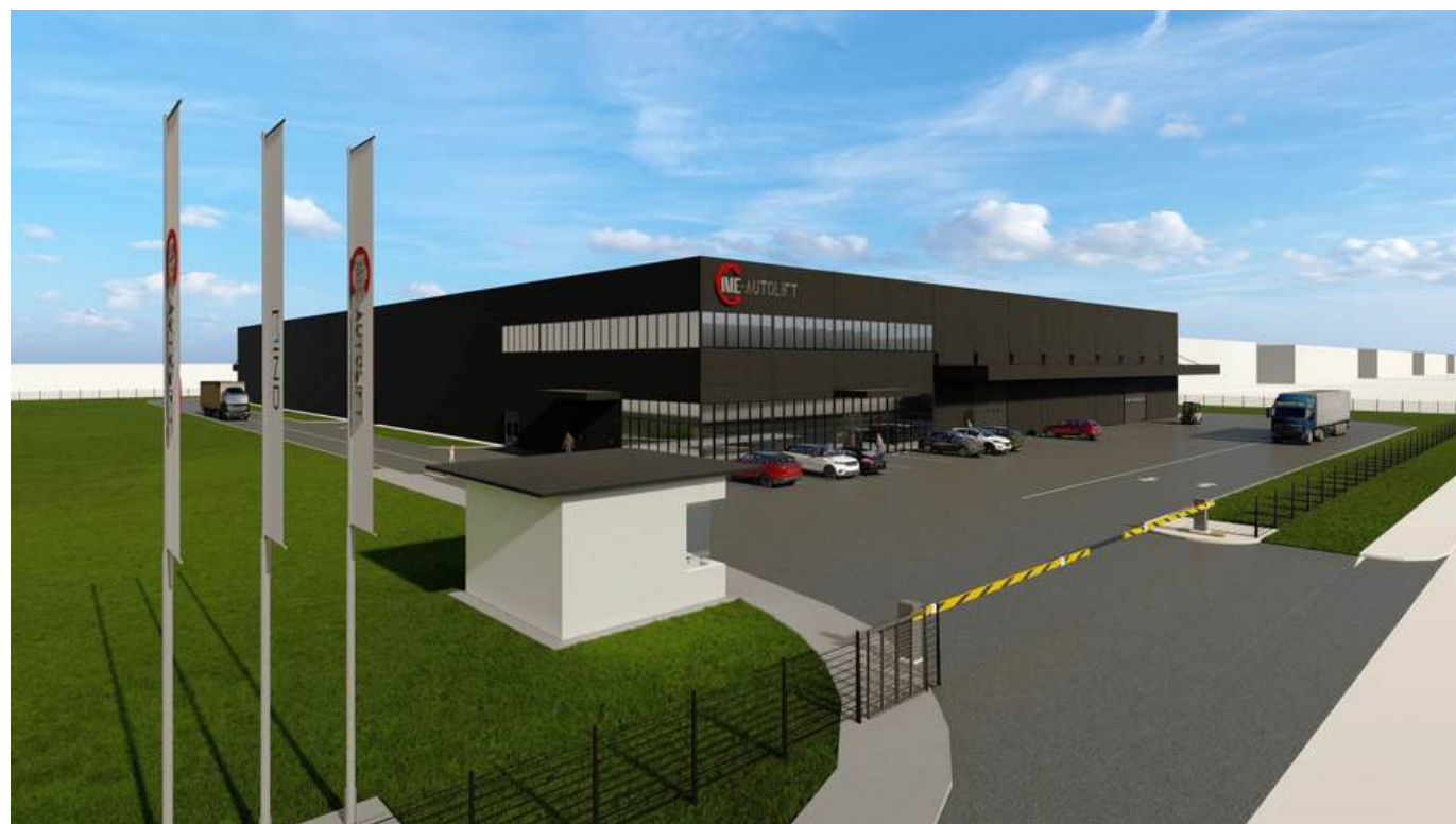
Production facility- IME-AUTOLIFT 2024- 2025
